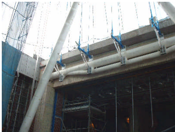
Figure 4. Lower anchorage to high level trusses
