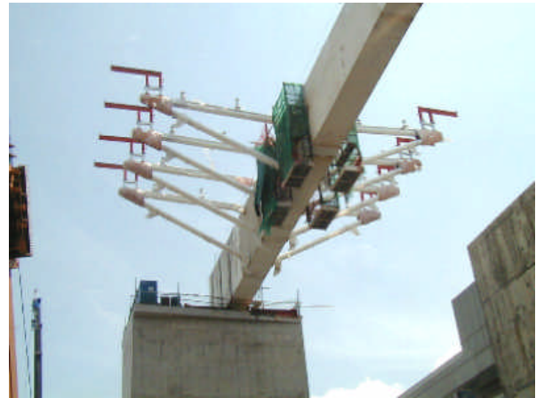
Figure 22. Installation of ribs
