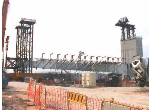
Figure 26. Lifting spine beam to its final level
