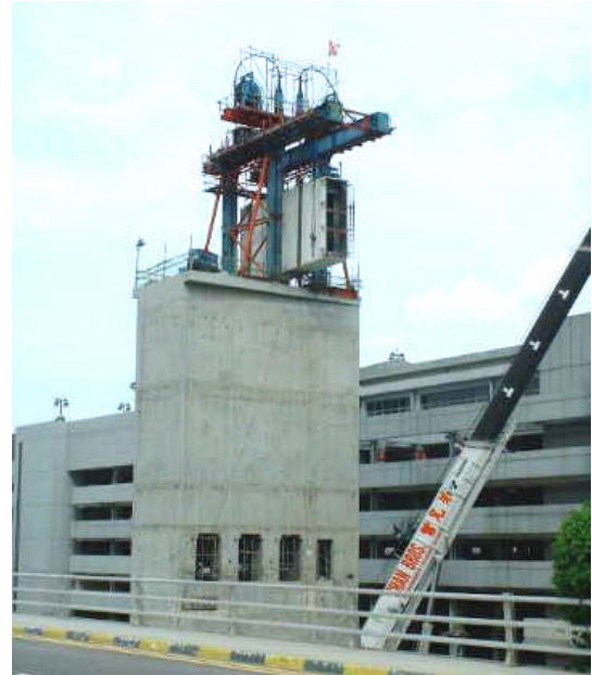
Figure 18. Erection of 1st module
