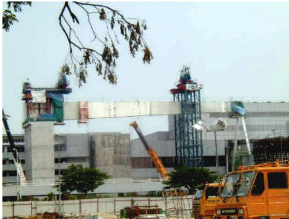
Figure 21. Terminal 2 spine beam erected.
