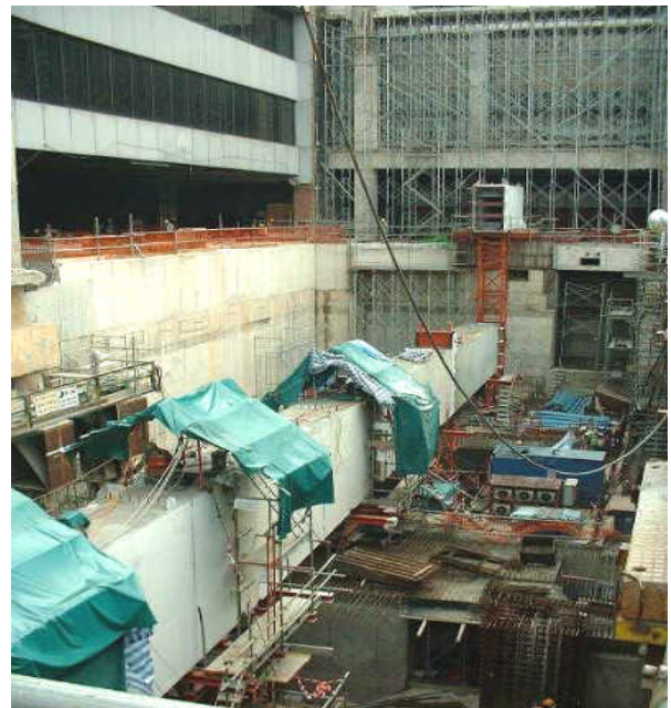
Figure 20. Modules 2 to 7 under assembly on temporary deck
