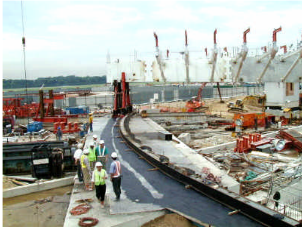
Figure 25. Sliding Terminal 3 spine beam.
